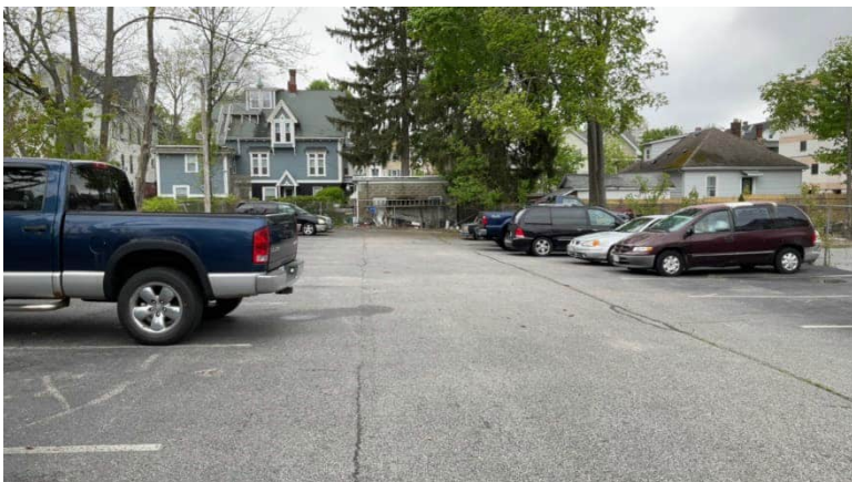
View of catchment for rear catch basin taken facing north.
