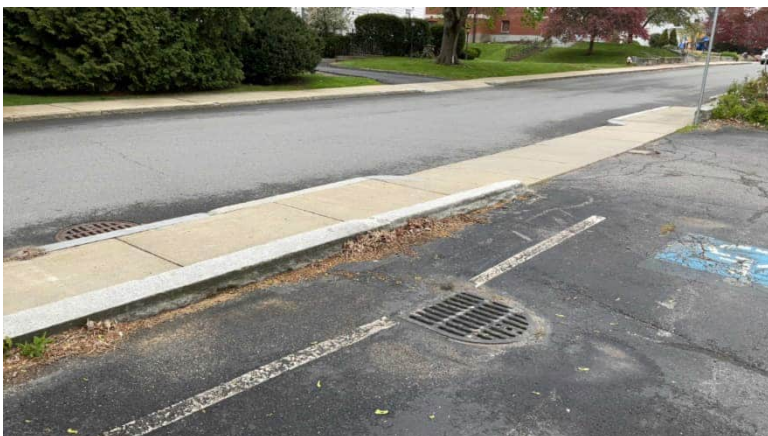
Existing catch basin at south end of parking lot outlets to stormwater infrastructure in the street.
