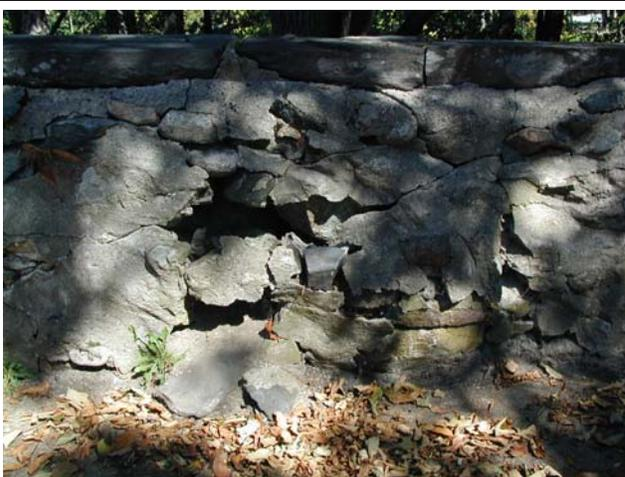
Figure 7. Example of wall failure. Note cracking and loss.
